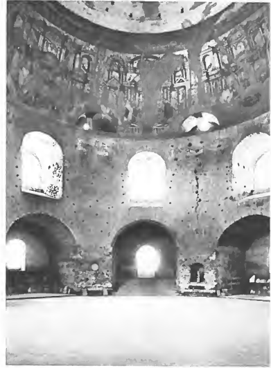
Interior of St George's church, Salonika, Greece, a fifth-century Byzantine round church whose geometry was based on the circle and the octagon. The nineteenth-century church of St George's, Tufnell Park, London, follows the same scheme.
