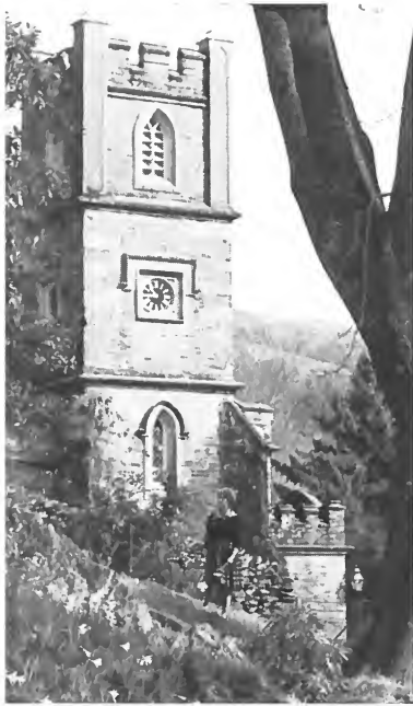
Rydal Chapel in Westmoreland (Cumbria), whose foundation in 1823 according to ancient geomantic usage is recorded in Wordsworth's poem, 'On seeing the foundation prepared for Rydal Chapel'.
