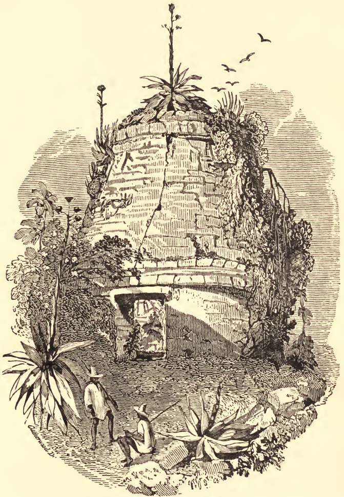
Fig. 35.—Circular Edifice at Mayapan.
