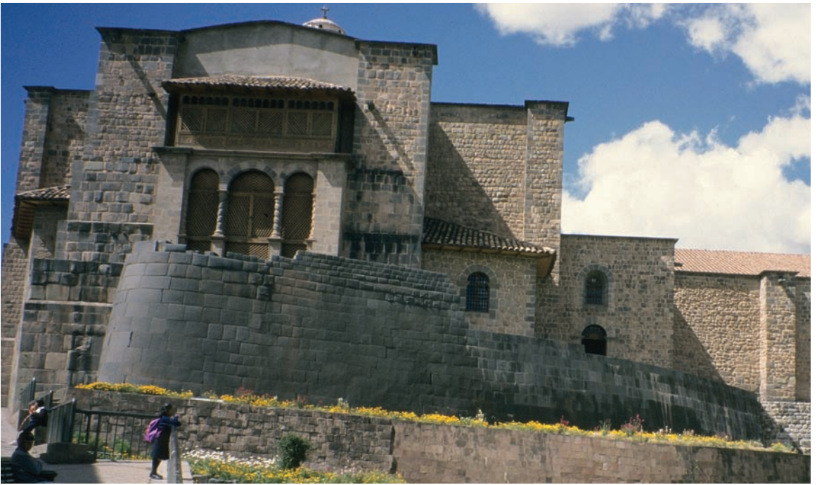
Figure 3.22. The elliptical wall of the Temple of the Sun (Coricancha) in Cuzco is one of the most astonishing examples of Inca stonework. The Dominican Church was constructed over the temple's remains.
