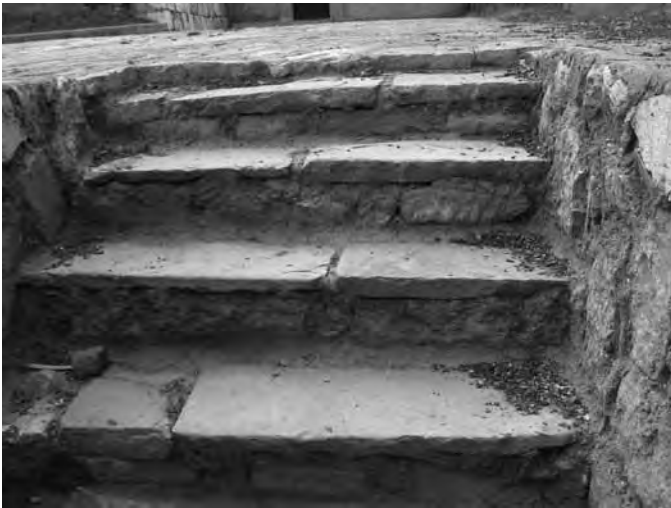
Figure 7.42. Uncarved red sandstone slabs in the main church in the plaza of Taraco.
