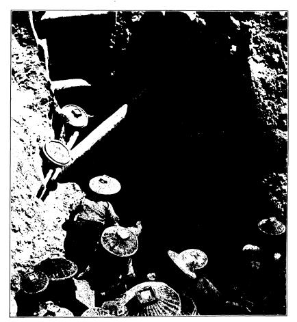
Fig. 2. Igorots stoping in Palidan slide. PLATE 21:
