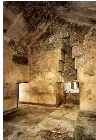
Figure 55 Entrance to the Queen's Chamber (right) and the corbelled niche in the eastern façade
