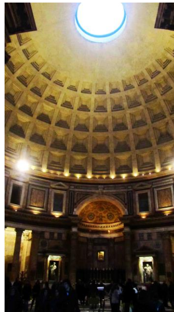
Figure 39 The view upon entering the Roman Pantheon showing the vertical qualities of the coffered dome with the central eye at the apex allowing controlled light from the heavens symbolizing the dome of the heavens
