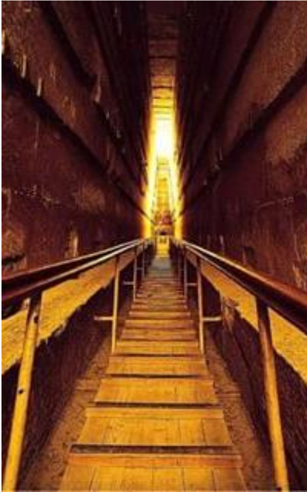
Figure 56 Image shows the interior space of the Grand Gallery with its corbeled walls inducing a sense of added height and accentuated ascension. ( https://upload.wikimedia.org/wikipedia/commons/thumb/d/d0/Cheops_grote_gallerij.jpg/170px-Cheops_grote_gallerij.jpg - visited: 2/11/2015 12:12 am)
